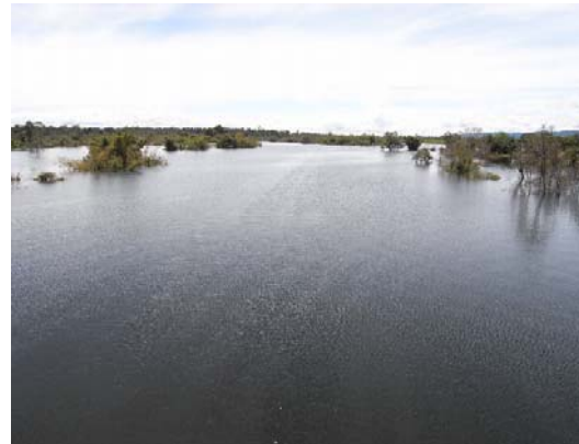
Trees left standing in the reservoir as it fills
