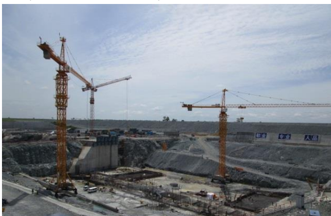
Lower Sesan 2 Dam under construction. (Photo taken on 27 th July 2015)
