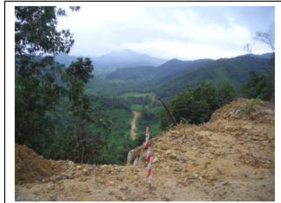
The road-link connecting Dawei SEZ planned area and Myanmar-Thai border. There are plans to expand this into a 4-lane highway. Railway, electricity links, oil and gas pipelines are planned to follow. (Photo: October 2015)
